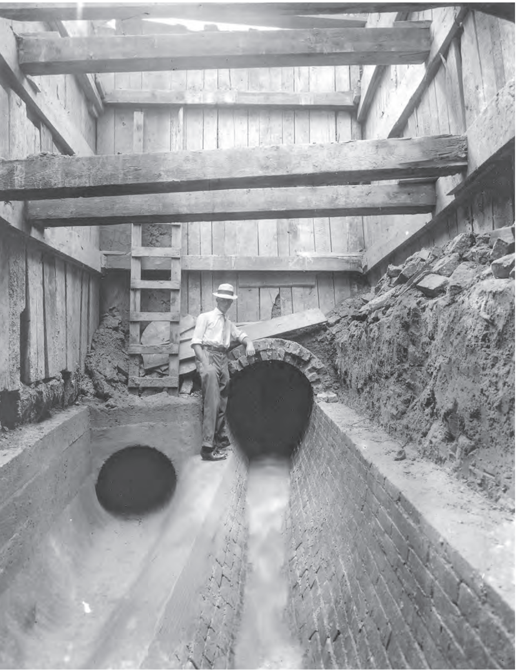
Taddle Creek, all piped up and flowing as part of Toronto's original sewer system.
